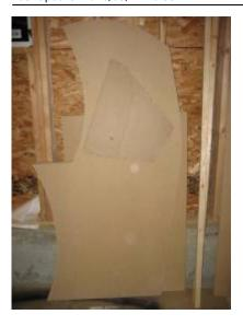
The top and back will be two pieces of curved plywood. Each piece will sit atop a brace frame that will connect it to the sides. The idea is for a flush outter shell that rides just lower than the Galaxian green T-molding along the edge, maybe 1/8".
