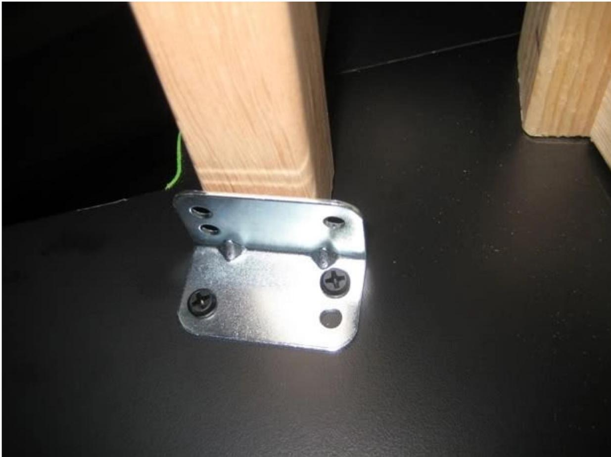
Here you can see there is exactly 1/4" of the L Shape sticking out beyond the bezel...perfect fit for the 1/4" plexi! (EDIT: Now using 1/4" glass).
