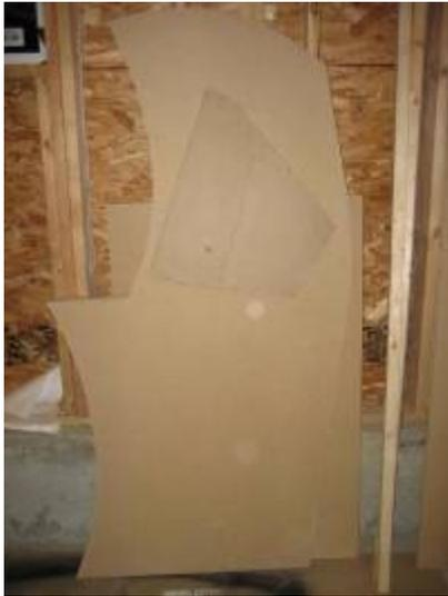
The top and back will be two pieces of curved plywood. Each piece will sit atop a brace frame that will connect it to the sides. The idea is for a flush outer shell that rides just lower than the Galaxian green T-molding along the edge, maybe 1/8".
