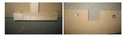
The top and back will be plywood. 1/8" on the top and 1/4" on the back. I will use one of the existing sides of the cabinet as a template for the curve of the exo-skeleton that the plywood will curve over. The back and top will each have 4 ribs. The outer side ribs of the top portion will connect to the sides of the cab via horizontal flanged inserts (the main horizontal support beams have vertical ones so this should be fine).
