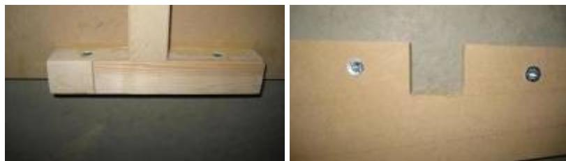
The top and back will be plywood. 1/8" on the top and 1/4" on the back. I will use one of the existing sides of the cabinet as a template for the curve of the exo-skeleton that the plywood will curve over. The back and top will each have 4 ribs. The outer side ribs of the top portion will connect to the sides of the cab via horizontal flanged inserts (the main horizontal support beams have vertical ones so this should be fine).
