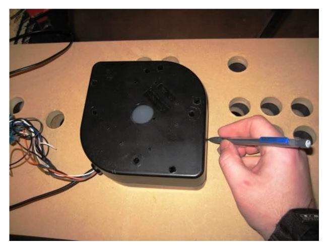
After tracing the mount I went back to my X Gaming CP to set the depth of my router. Both CP's are 5/8". I prefer this size for a CP when using laminate as it's easy have the T molding cover flush the edge of the laminate. Using 5/8" CP I will route the Trackball recess to 1/4" of MDF left:
